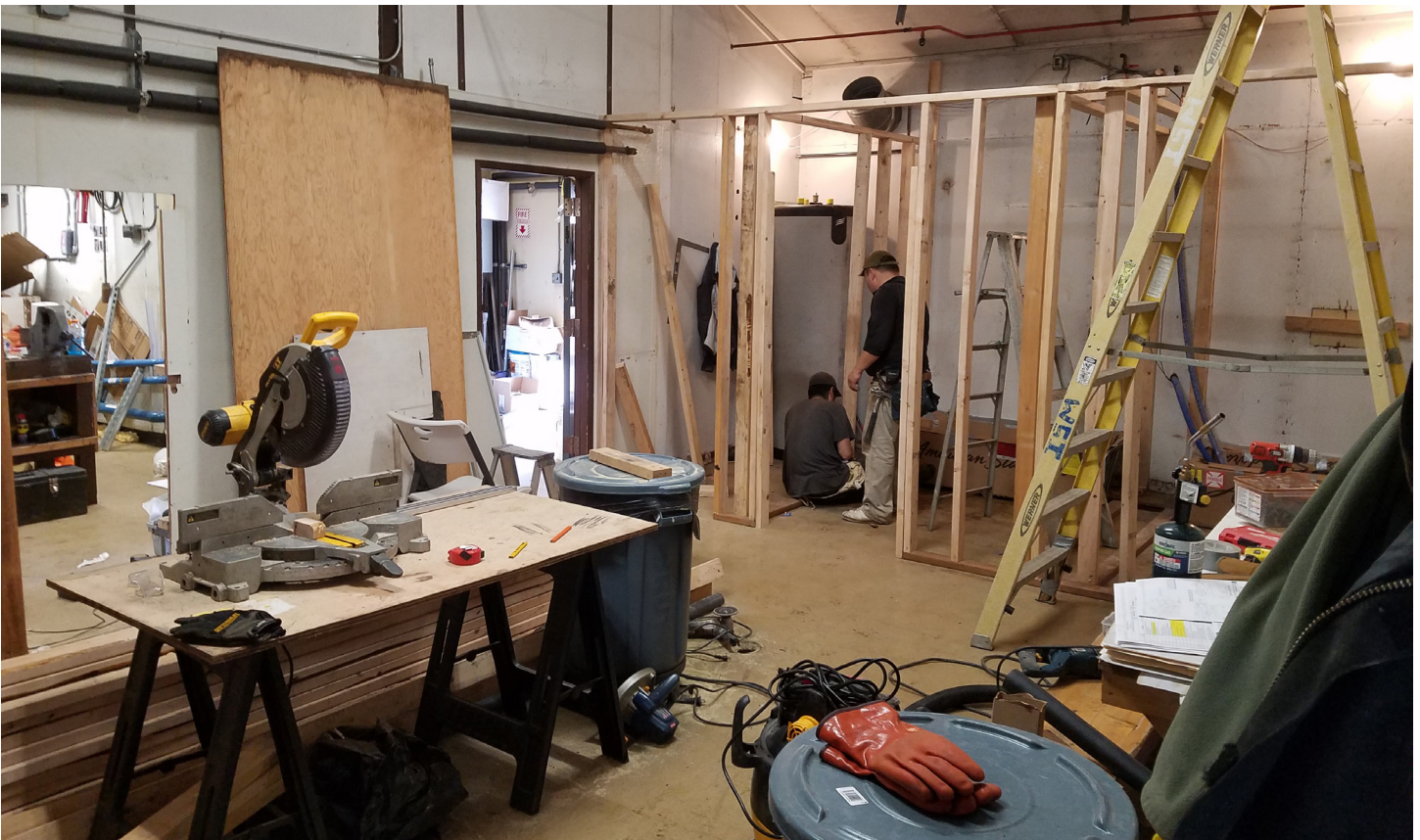
ANTHC employee, Martin Wortman, and a local hire from Newtok work on the Washeteria renovation.
