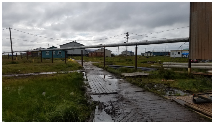
Broken and sinking boardwalks are prone to flooding and make it hard for community members to transport belongings in Newtok.
