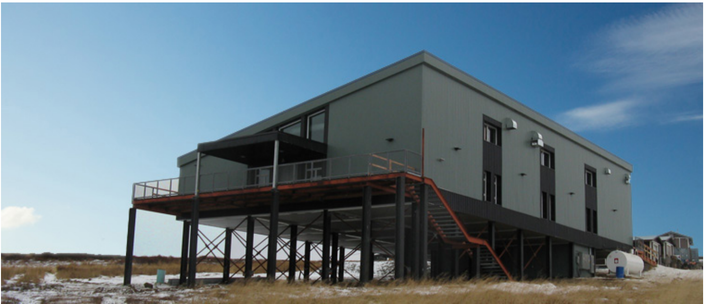
UICC will construct the interior of the MEC to accommodate school service starting this October.
